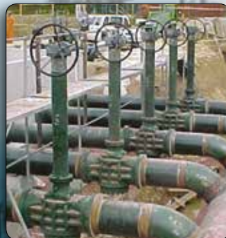
Client: SNAMPROGETTI Location: LOSTORF (CH) Valve: 20" Cl. 600 Venturi with Stem Extension.
