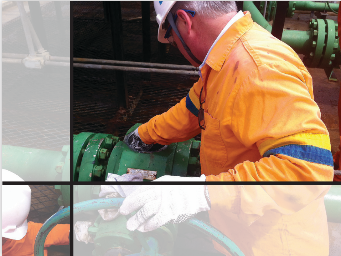
Training on site and Field Commissioning
